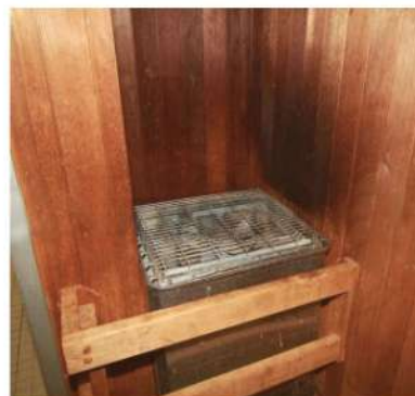
Example heat damage behind sauna heater
